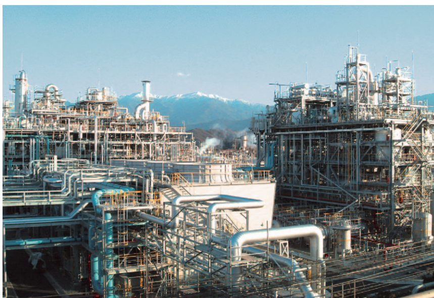
Figure 5. Ammonium sulfate-free \epsilon -caprolactam plant based on ammoxidation and vapor-phase Beckmann rearrangement (2003, Sumitomo Chemical Co., Ltd).
